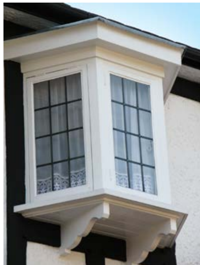
Figure 18: Window details at Sudbury Court
