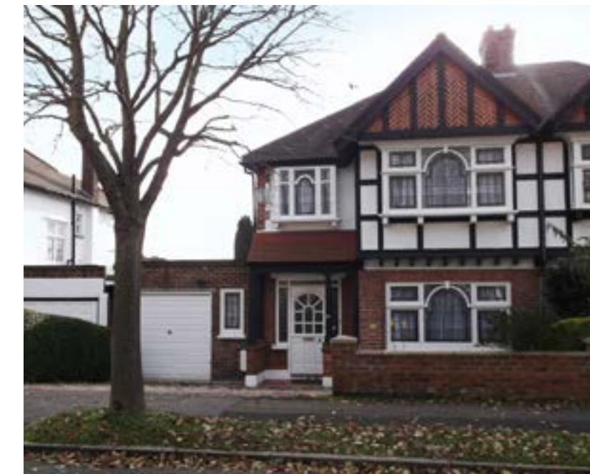
Figure 22: Decorative features at Sudbury Court
