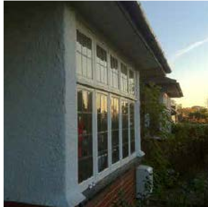
Figure 17: Window details at Sudbury Court
