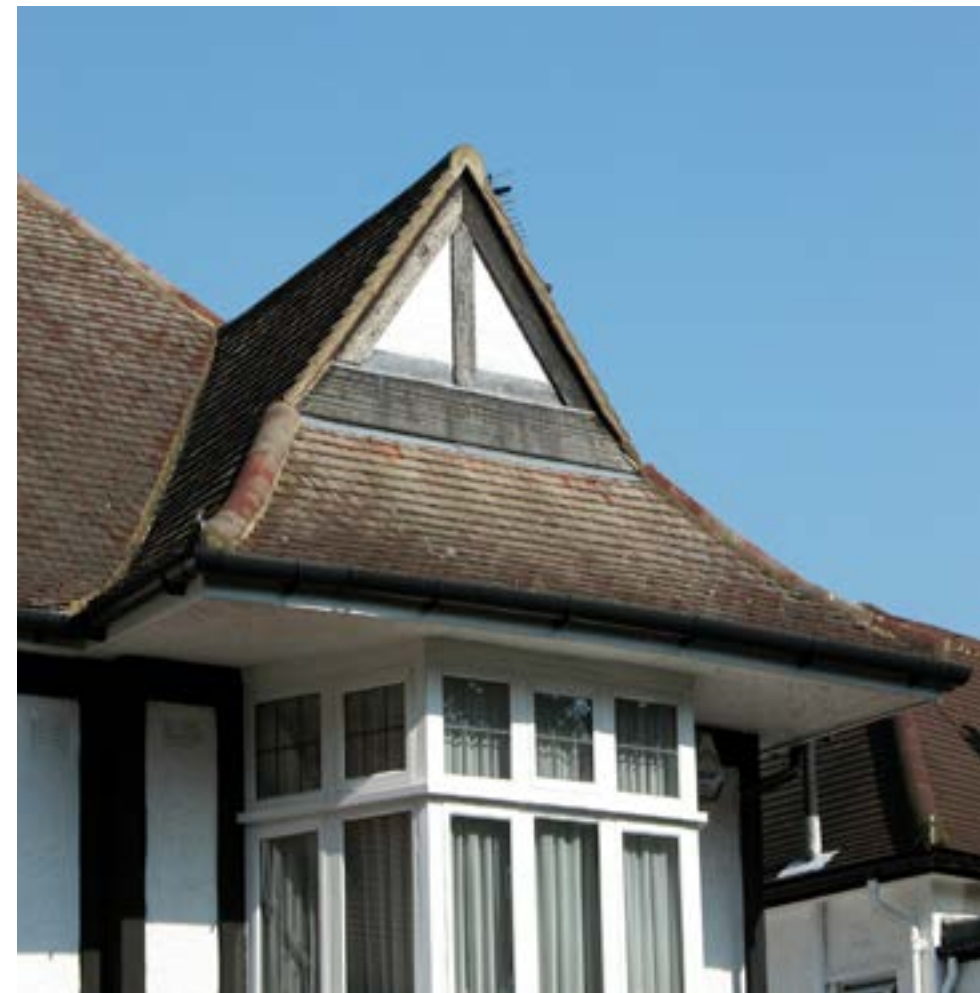
Figure 19: Window details at Sudbury Court
