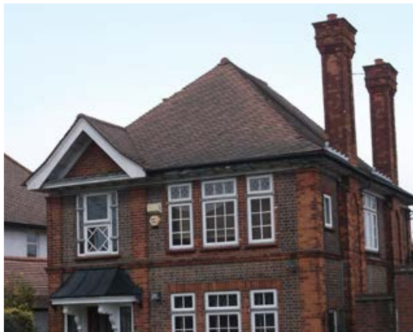
Figure 26: Decorative brick chimney at Sudbury Court
